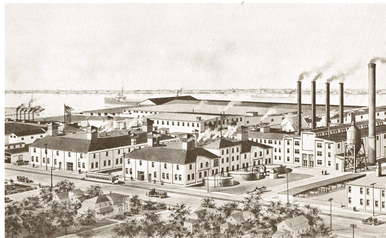
(Below) The Diamond Crystal plant in 1919.
